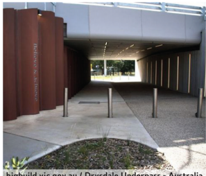
bigbuild.vic.gov.au / Drysdale Underpass - Australia
