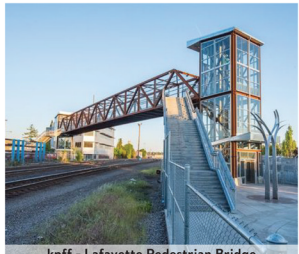
kpff - Lafayette Pedestrian Bridge
